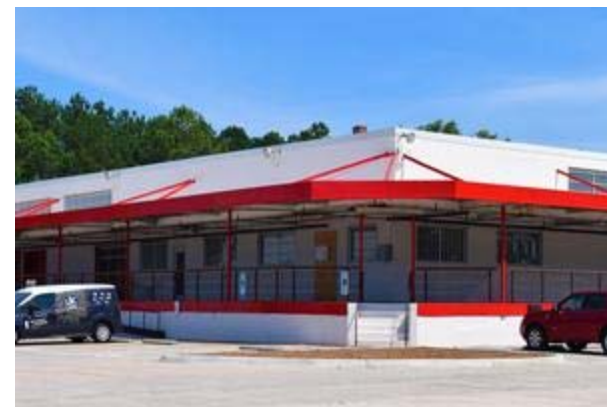
An "after" photo of the Dock 1053 warehouse building, home to Lynwood Brewing Concern and multiple other businesses.
