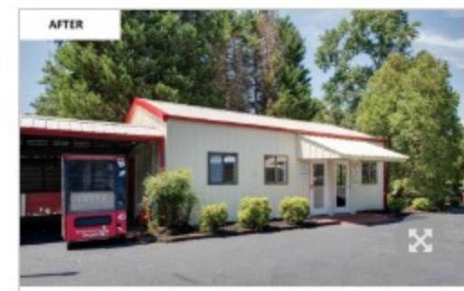
Office Exterior- Post-Renovations
